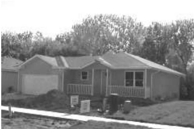
A completed house by Northeast residential construction class
